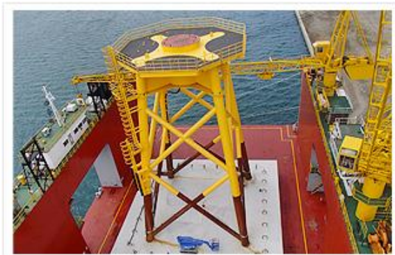
Fig 1 Example of Jacket Foundation [3]
